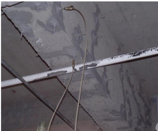
After filling the cracks to rejection, above, the material is cured, it will create a bond that exceed the strength of the original substrate. Once cure the supply tubing is removed and the process is completed.
