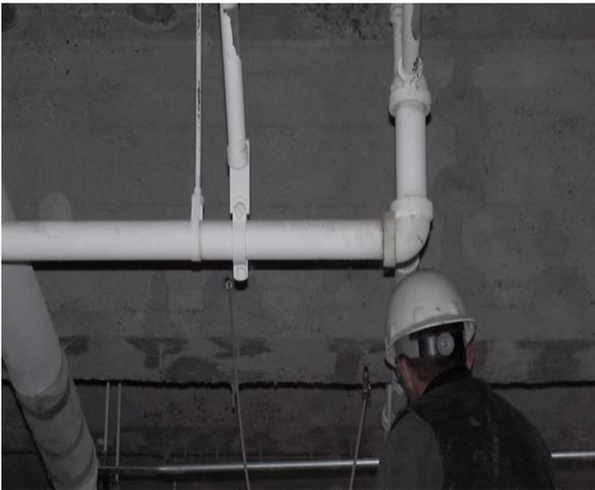
Setting up the Pro-Seal Power Kote Injection Grade induction ports, above. The Power Kote Injection Grade plural component medium will be pumped deep into the concrete to heal structural cracks and other cracks in the concrete mass.
