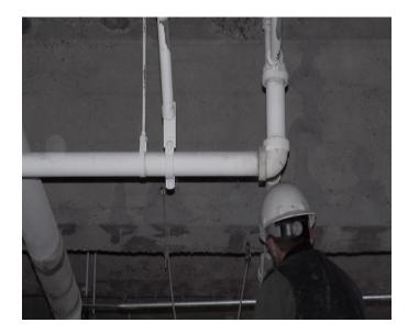
Setting up the Pro-Seal Power Kote Injection Grade induction ports, above. The Power Kote Injection Grade plural component medium will be pumped deep into the concrete to heel structural cracks and other cracks in the concrete mass.
