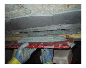
Utility tunnel at LA Trade Tech. The concrete is carbonizing, and the rebar is nearly completely oxidized. This is not inly making the tunnel a safety hazard but also the east wall of a multistory building directly over the longitude of the tunnel could collapse into the failed tunnel.
