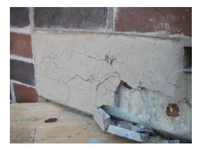
Exterior concrete building facade trim on Wilshire Blvd, shrinking, cracking breaking up and falling onto the sidewalk below. This is creating a tremendous liability and safety hazard. Solution Pro-Seal PowerPatch Flexible®.
