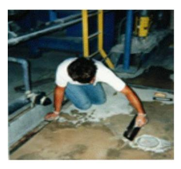
Patching and leveling concrete damaged by acids in a pickling plant With Pro-Seal Power Patch.
