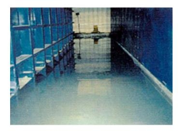
The finished floor, Pro-Seal Power patch was used to heal and level the floor through wet acids. Pro-Seal PP/PK primer was used to create a primed base for the Pro-Seal Power Kote III build up coats. The Pro-seal PowerKote build up base was top coated with Pro-Seal PP/PK type III, a highly chemical resistant topcoat as the final coats.
