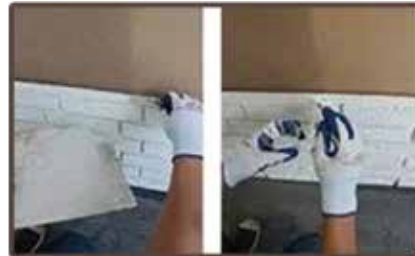
6. Caulking, repairing, cleaning
