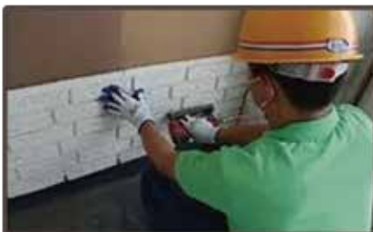
5. Reinforced with gun nails
