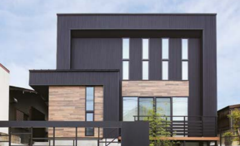
Exterior and facades
