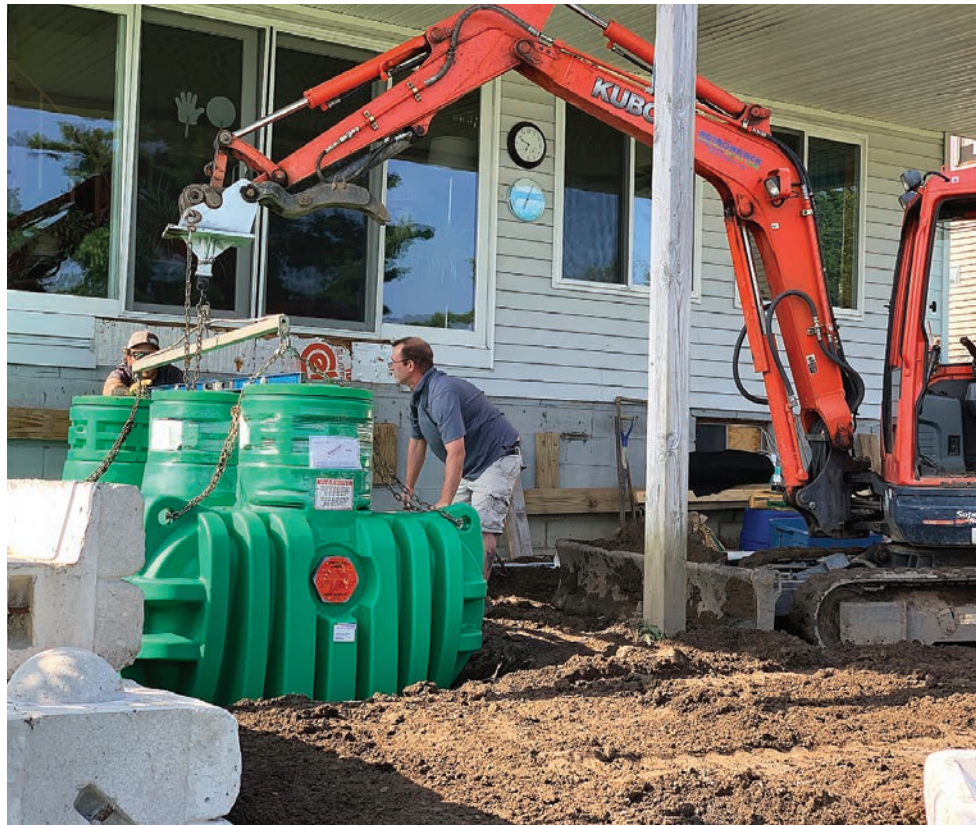
▲ The new Singlair treatment tank is lowered into its hole at the house on Great Sacandaga Lake by Zielinski, left, and Gifford, right. Because the porch roof was not removed, operators had to be particularly careful when swinging the Kubota mini-excavator.
