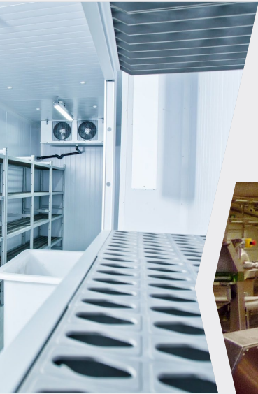
Cold storage cells (0 °C / +8 °C) Blast chilling cells
