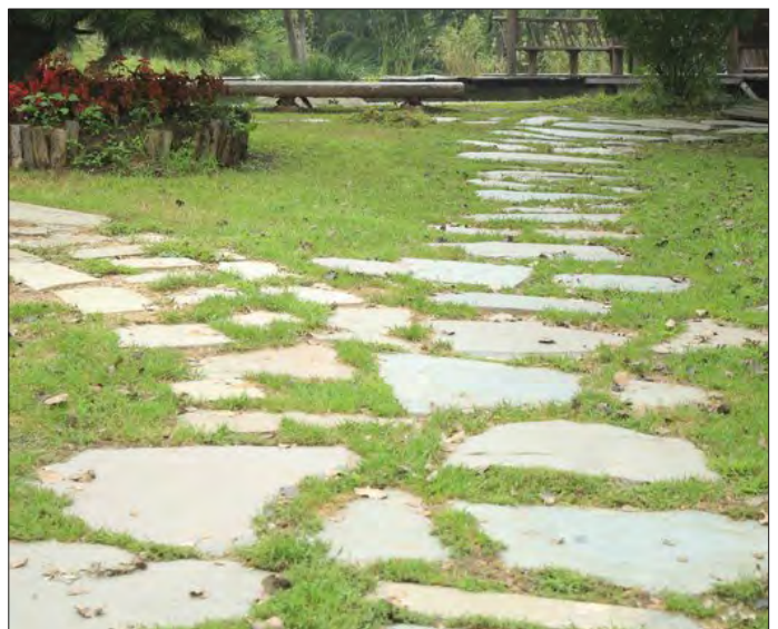
Figure 35. Flagstone pavers installed at ground level
