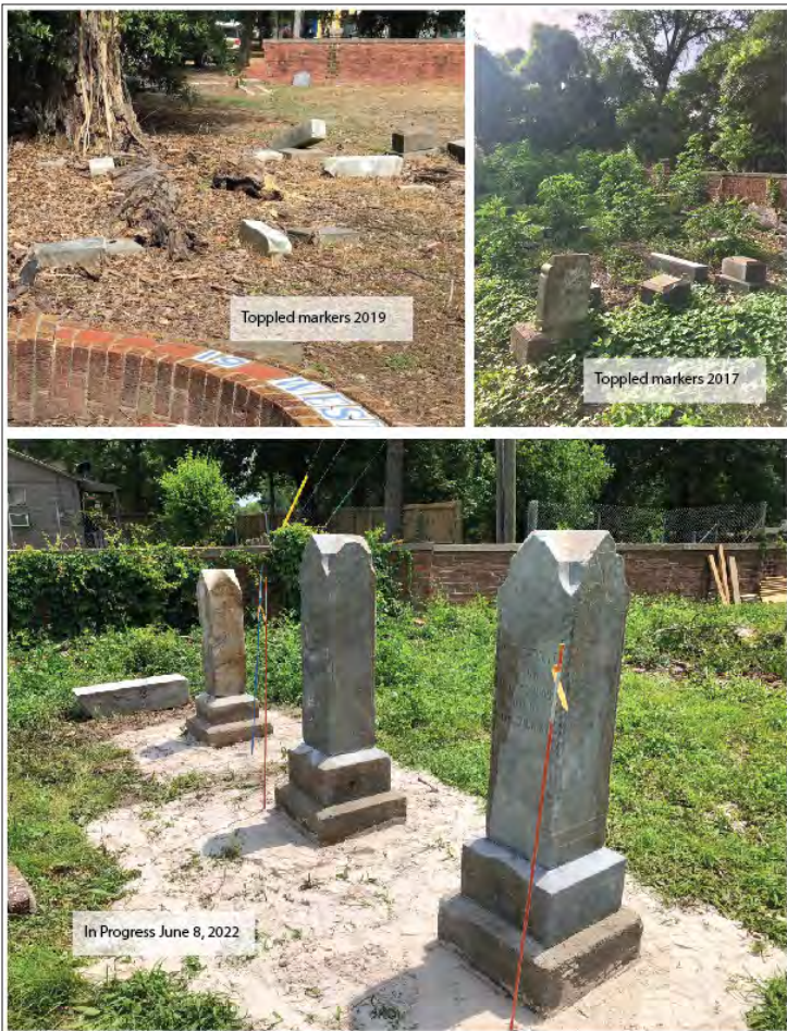
Figure 14. Examples of grave markers before and after resetting and repairs in 2022 (WCA, McDoux)
