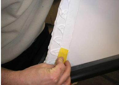
Squeeze a few beads of 4/5200 adhesive along the length of the bumper (3/8" diameter) as well as on the hull. Spread out the beads from center to the edges, ensuring the 4/5200 layer is thickest in the center. Apply a single bead to the center of the bow area and spread it out to the pencil markings Check both 4/5200 layers for trapped bubbles after spreading, and spread them out as necessary
