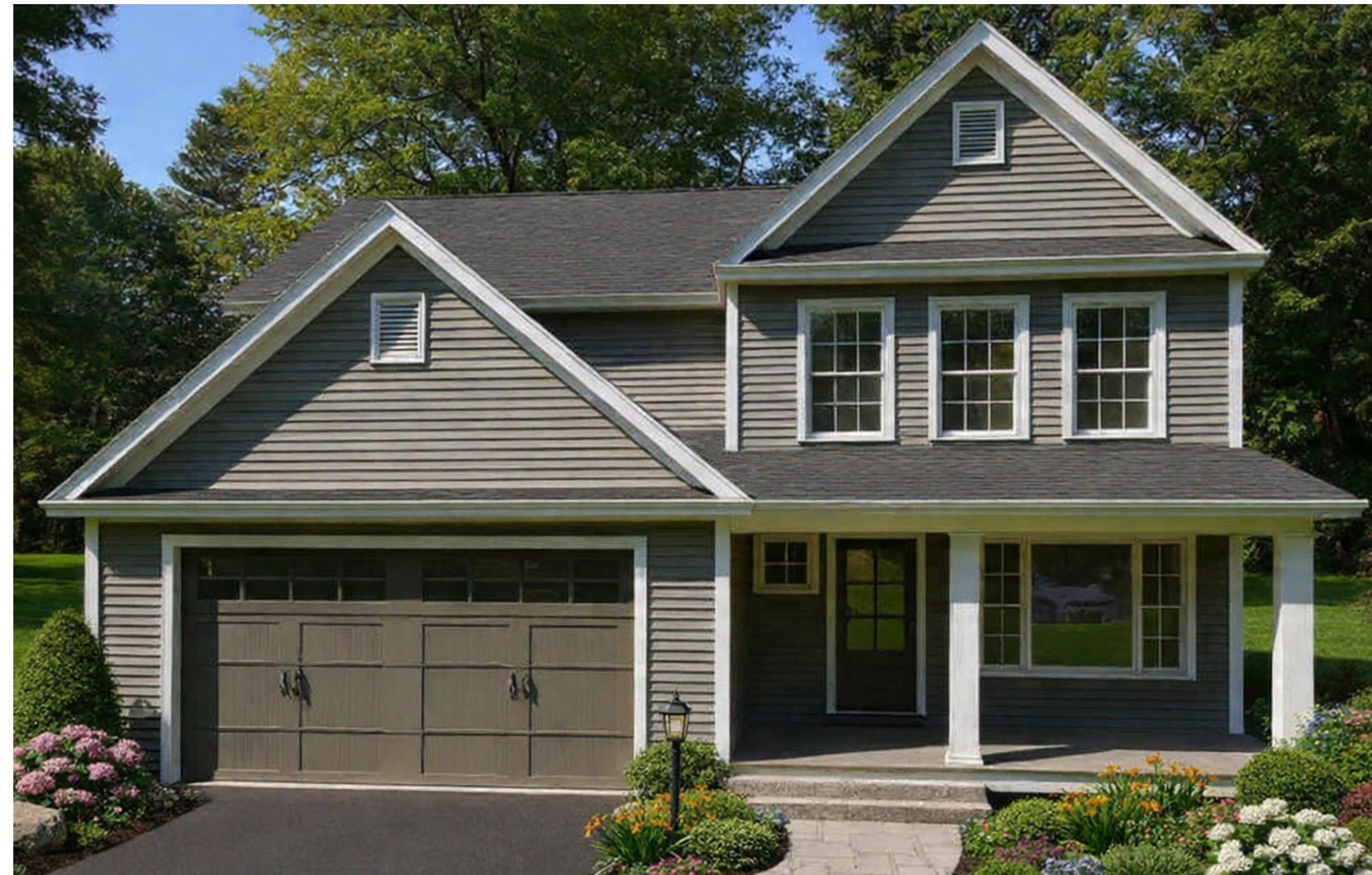
NEW HAMPSHIRE DEVELOPMENT GROUP COLONIAL 2 PLAN CANTERBURY PROJECT 114 WEST RD CANTERBURY, NH
