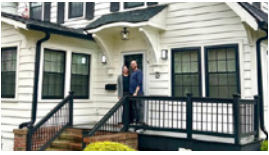
82 Oakview Ave, Maplewood
