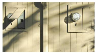
At left are electric meters for adjacent condos located at the rear of some the older condominiums. Some of the older condos have meters in front by the kitchen window. The little lever shown on right of the meter is lifted to expose the master circuit breaker for the condo. Individual circuits are located inside the house and could also be used if accessible during an emergency.
