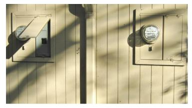
At left are electric meters for adjacent condos located at the rear of some the older condominiums. Some of the older condos have meters in front by the kitchen window. The little lever shown on right of the meter is lifted to expose the master circuit breaker for the condo. Individual circuits are located inside the house and could also be used if accessible during an emergency.
