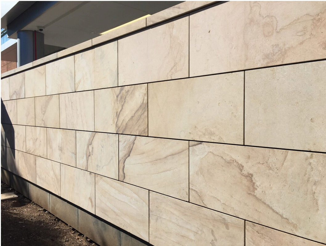
Retaining walls for large and smaller projects.
