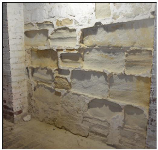
The above photo shows how the humidity has damaged the original sandstone walls, deterioration can be seen in the accumulation of sand at the base of the wall.
