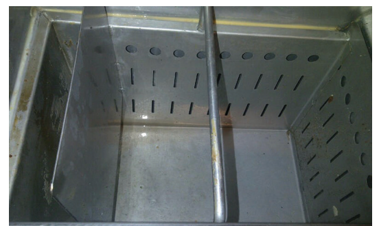
AFTER: Clean Grease Trap
