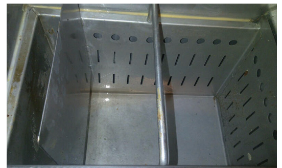
AFTER: Clean Grease Trap
