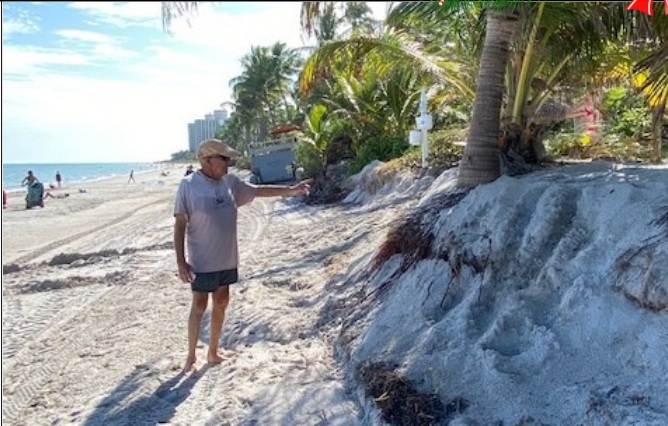
Member Doug Biggers points out beach erosion
