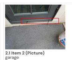
(2) Stain used to protect main doors has faded or failed, and need prep and stain again.
