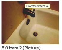
(2) The diverter on tub spout does not divert all water from tub to shower enough to affect the flow.
