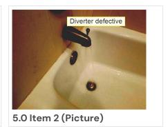
(2) The diverter on tub spout does not divert all water from tub to shower enough to affect the flow.
