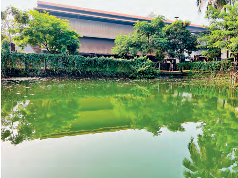
Rainwater harvesting facility at Peekay Calicut which is having a capacity of 1183 M3
