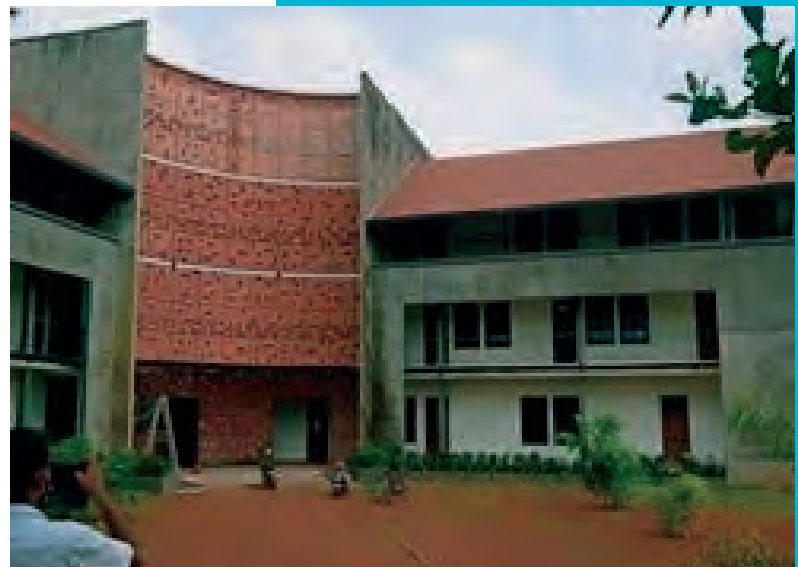
A most modern physics block has been built by Peekay Steel and handed over to Farook College. Farook College is a government-aided, autonomous arts and science college located in Feroke, near Calicut, Kerala.
