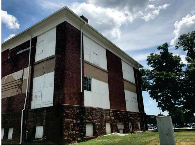
Photo 7: Exterior View of Bennet Building [Looking toward Northwestern Corner]
