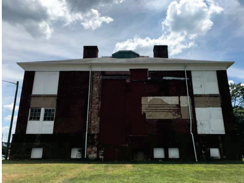
Photo 6: Exterior View of Bennet Building [Looking toward Northern Face]
