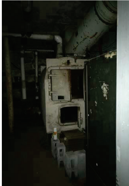
Photo 14: Boiler Room [North End of Basement]
