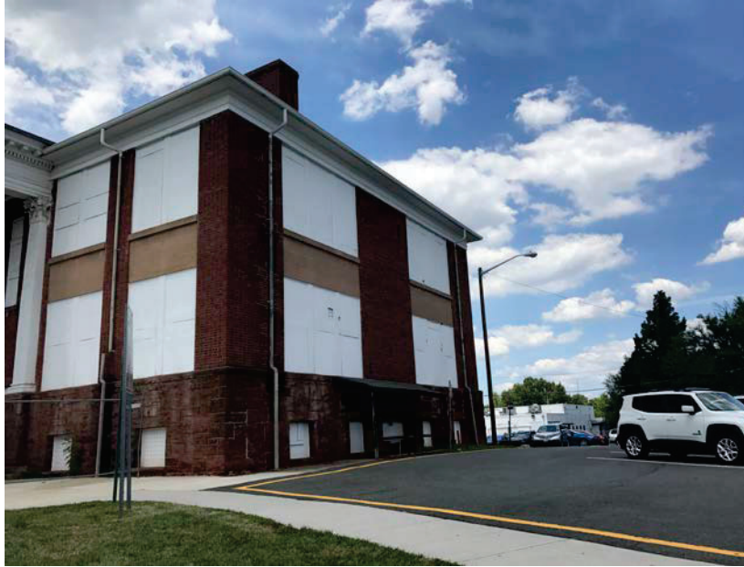
Photo 3: Exterior View of Bennet Building [Looking toward Southeastern Corner]
