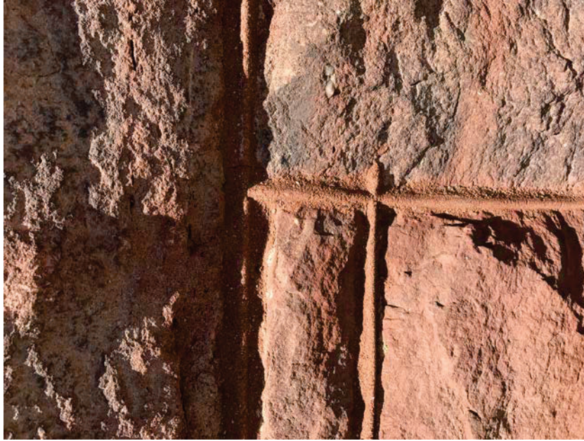
Photo 17: HA17 Exterior red brick mortar on the exterior of the subject property (B47-B49)
