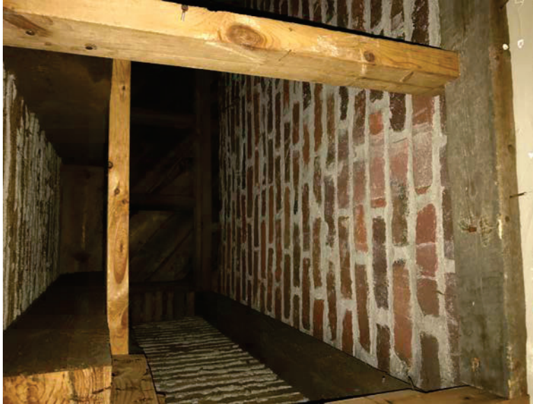
Photo 21: Planking under Hardwood Flooring
