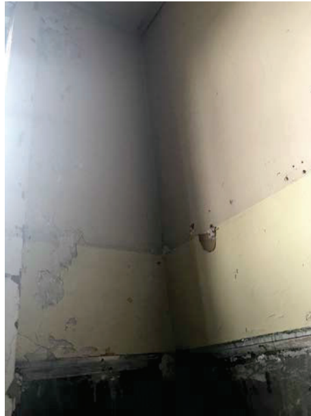
Photo 5: Cream and beige paint on the plaster walls throughout the classrooms on the 1 st floor
