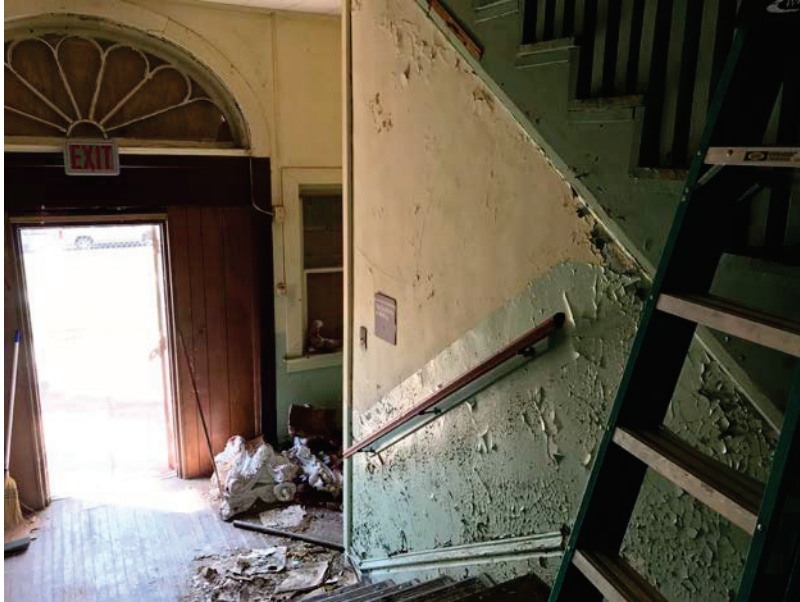
Photo 10: Entryway/Front Door [Looking towards Southwest]
