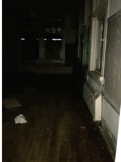
Photo 6: White paint on the plaster walls throughout the classrooms on the 1 st floor
