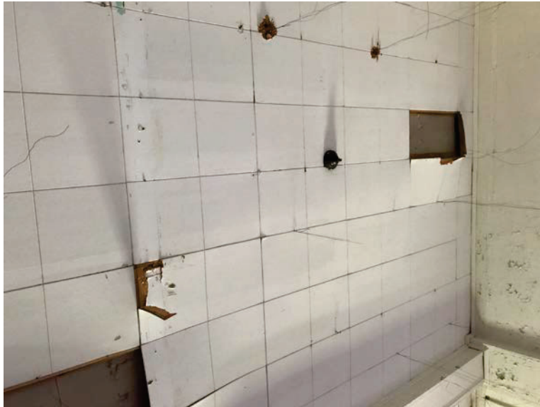
Photo 23: 14" x 14" Ceiling Tiles [1 st Floor]
