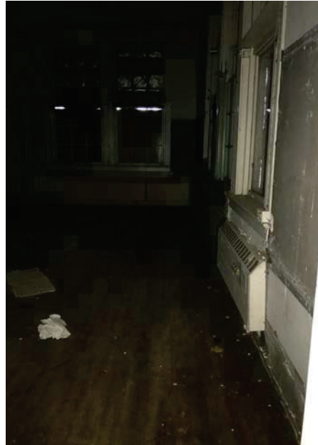
Photo 12: Classroom [1 st Floor, 1 st room on left]
