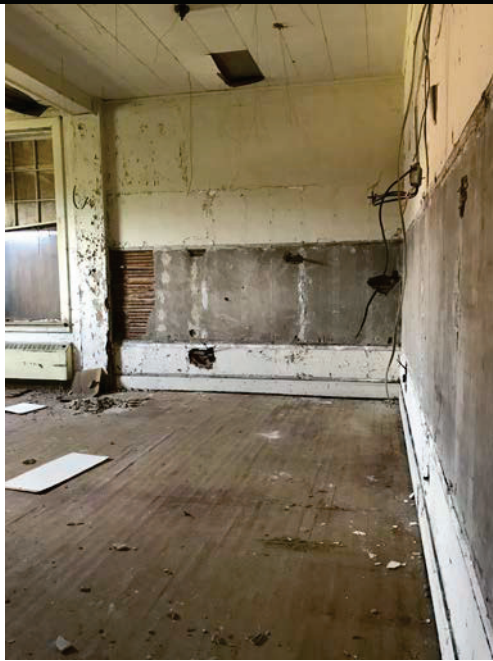
Photo 13: Classroom [1 st floor, 2 nd room on left]
