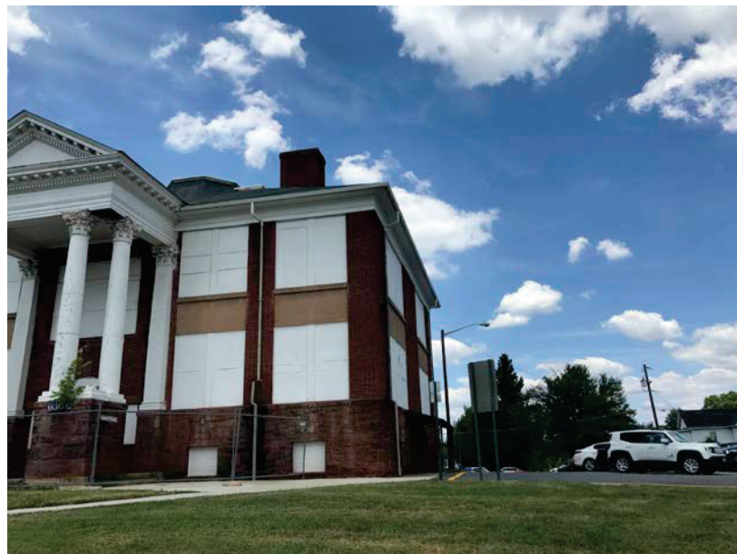
Photo 2: Exterior View of Bennet Building [Looking toward Southeastern Corner]
