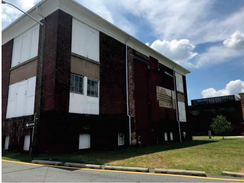
Photo 5: Exterior View of Bennet Building [Looking toward Northern Face]
