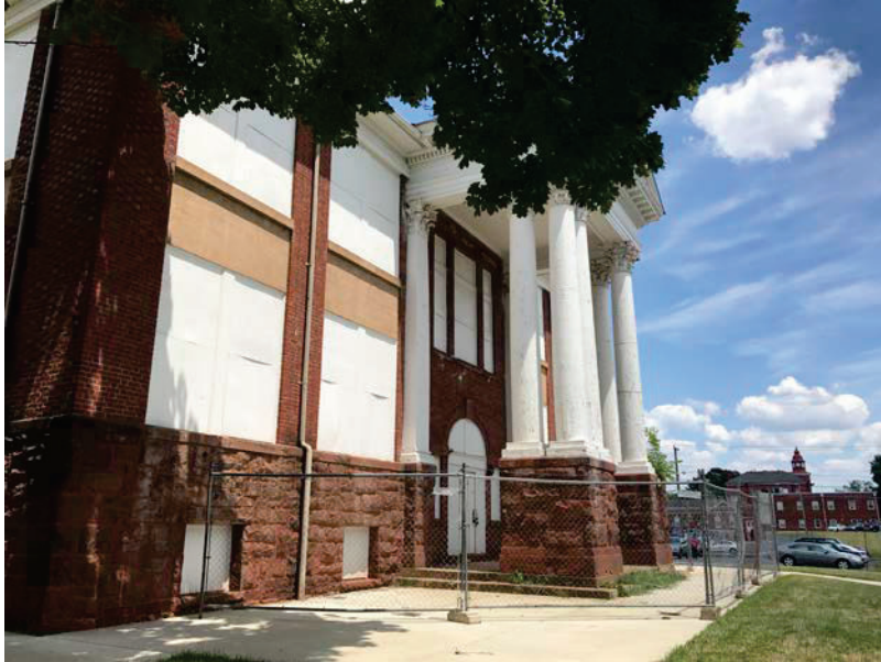
Photo 8: Exterior View of Bennet Building [Looking toward Southwestern Corner]
