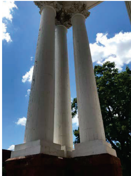
Photo 8: HA8 Exterior columns at the front entrance (B22-B24)
