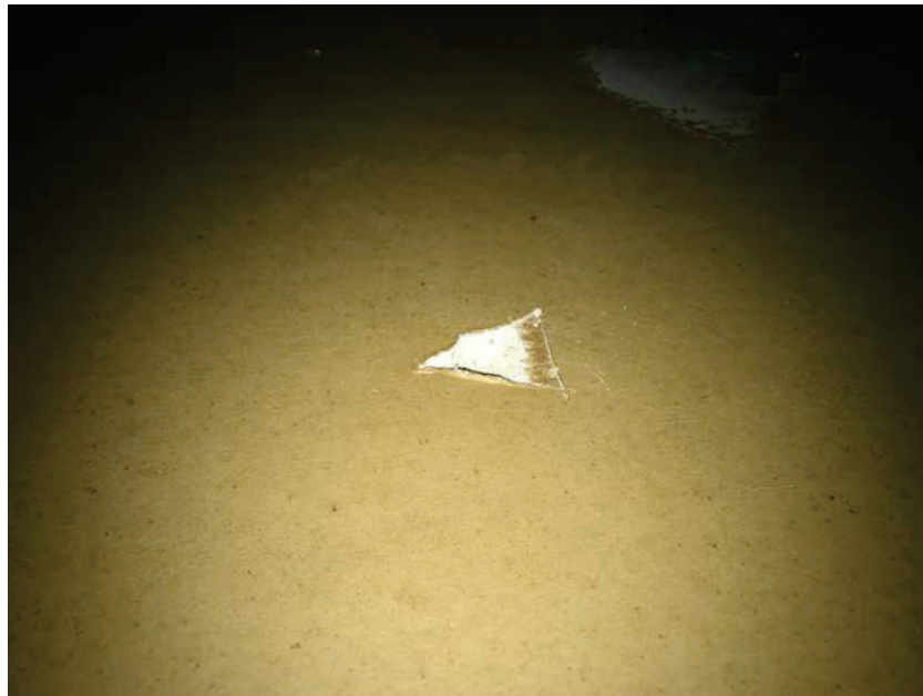
Photo 3: HA3 Drywall located throughout the subject property (B07-B09)
