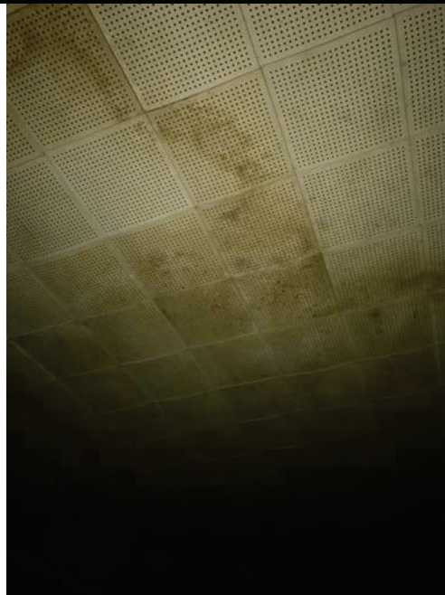
Photo 14: HA14 12"x12" cork ceiling tiles in the basement classrooms (B40-B41)
