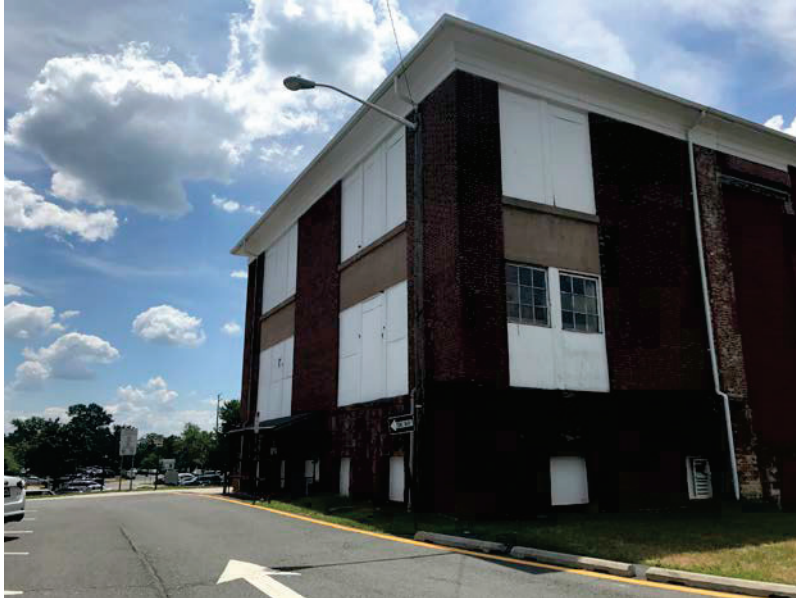
Photo 4: Exterior View of Bennet Building [Looking toward Northeastern Corner]
