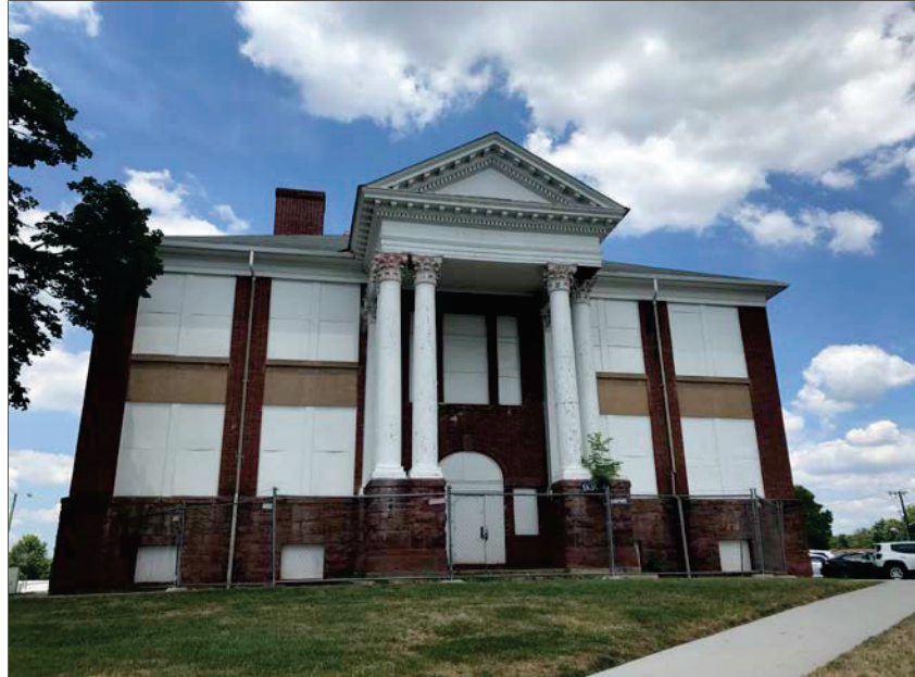
Photo 1: Exterior View of Bennet Building [Looking toward Southern face]
