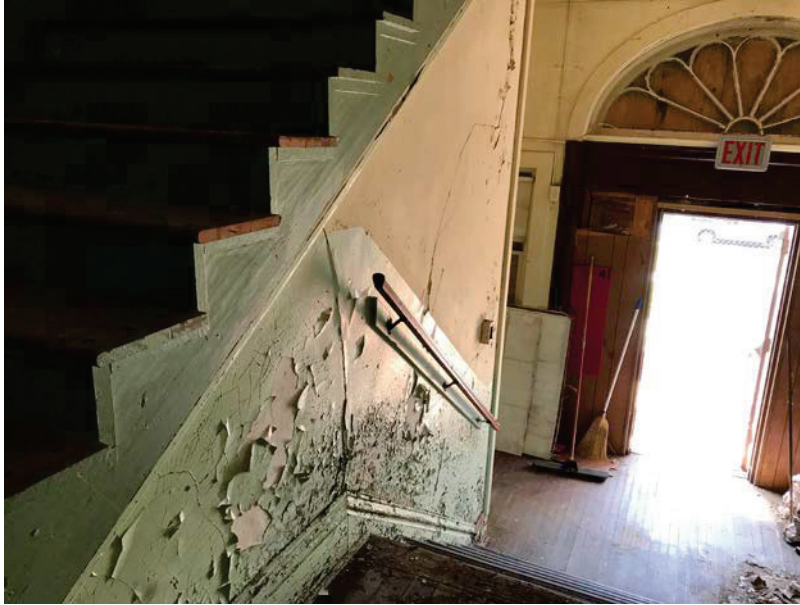
Photo 9: Entryway/Front Door [Looking towards Southeast]
