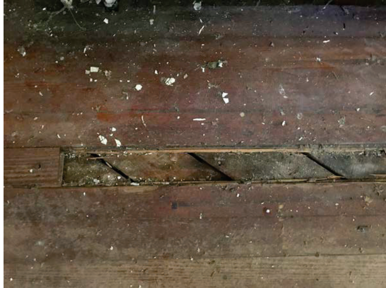
Photo 22: Closeup of Planking under Flooring
