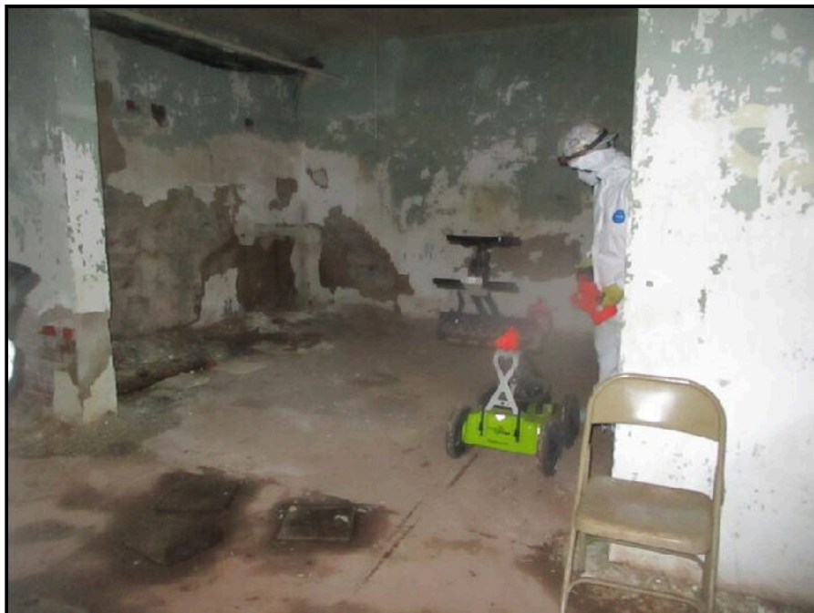
Photo showing a potential anomaly marked during the GPR survey in the basement of the Bennett Building.
