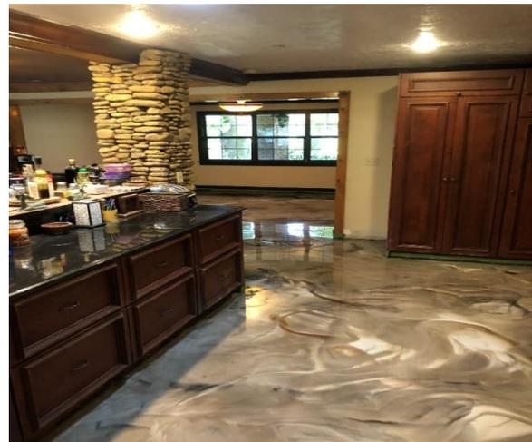
Floor was primed with black Moisture Mitigating Epoxy. Then 55 sq. ft per gallon of Tru-Flow 3D Metallic Epoxy was applied using pearl & cappuccino metallic pigments. The black base coat gave this floor a third color dimension since metallic pigments are translucent.
