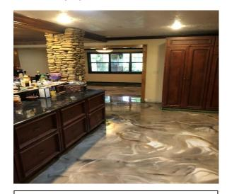
Floor was primed with black Moisture Mitigating Epoxy. Then 55 sq. ft per gallon of Tru-Flow 3D Metallic Epoxy was applied using pearl & cappuccino metallic pigments. The black base coat gave this floor a third color dimension since metallic pigments are translucent.
