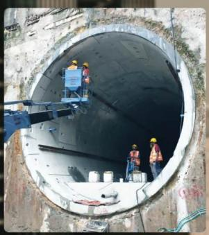
One of the job scope done for this project is drilling holes and preparing injection packer staggered along the leaking points, sealing of the leakage at tunnel segment with low-viscosity and injected grout and subsequently patch surface crack points and removal of packer.
