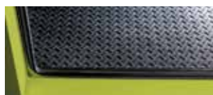
Container floor with crosshatch metal pattern surface
