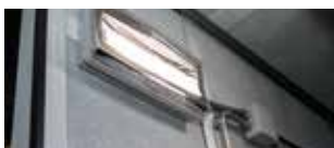
Internal lighting system
