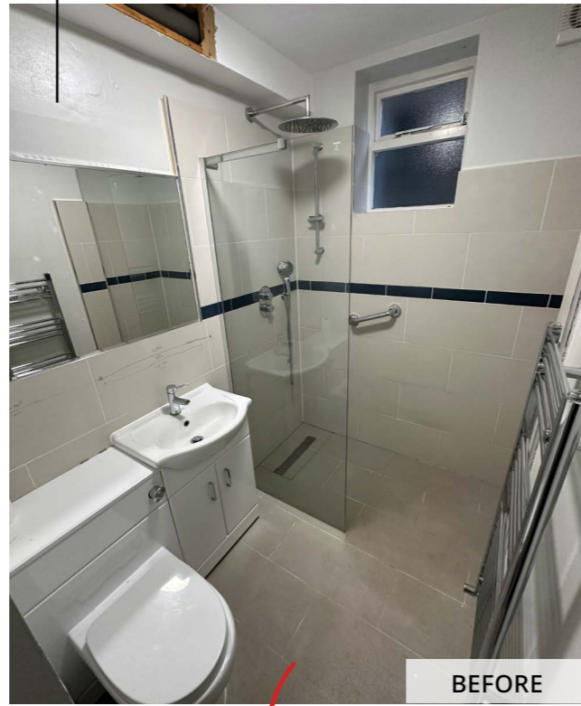
North London, NW5 Bathroom Installation
