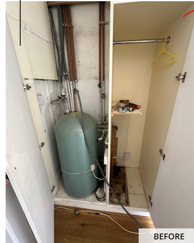
London, SW6 | Hot Water Cylinder Replacement
