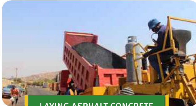
LAYING ASPHALT CONCRETE
