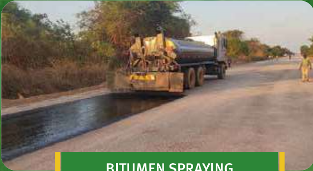
BITUMEN SPRAYING
