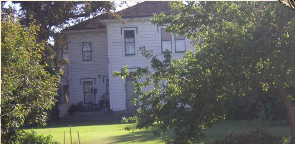
Duncan home today, built 1879 -- site of many early pioneer picnics in its surrounding Thousand Oaks area
