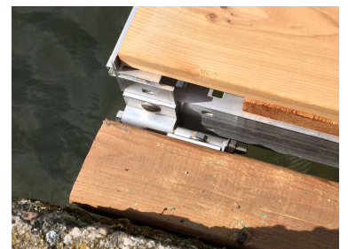
Ramp to Shore Hinge
