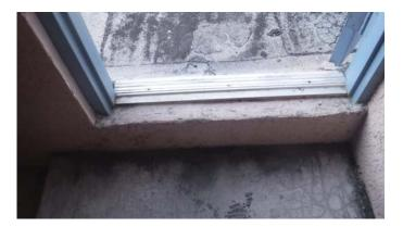
Mechanically fastened flashing
