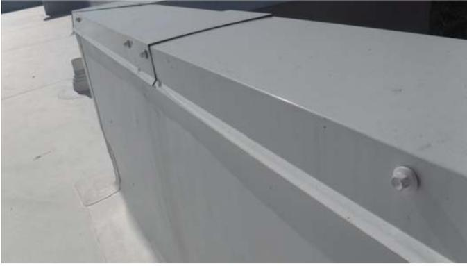
Mechanically fastened flashing
