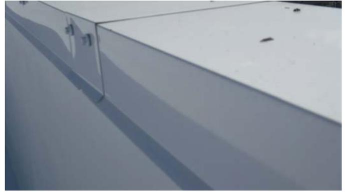
Mechanically fastened flashing
