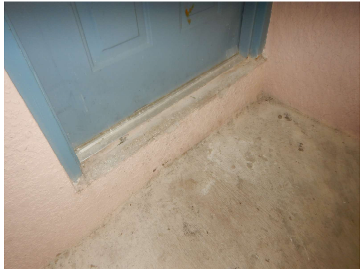
Concrete roof deck
