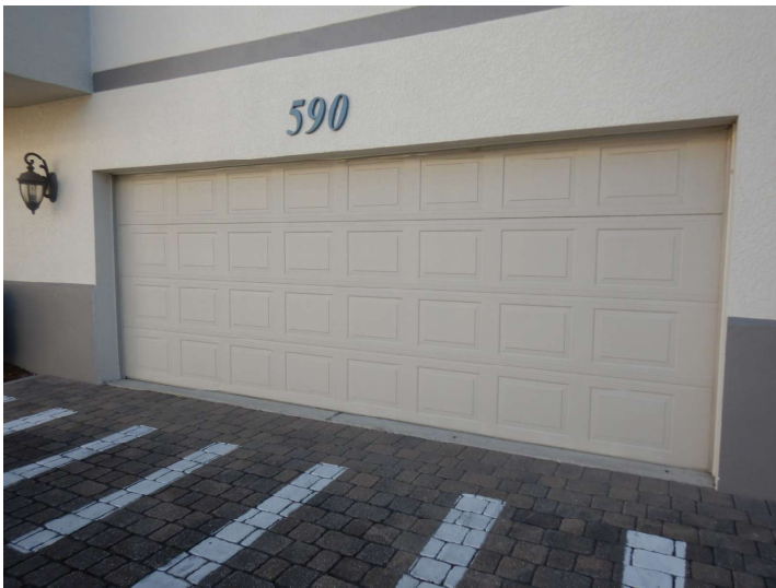
Non glazed garage opening
