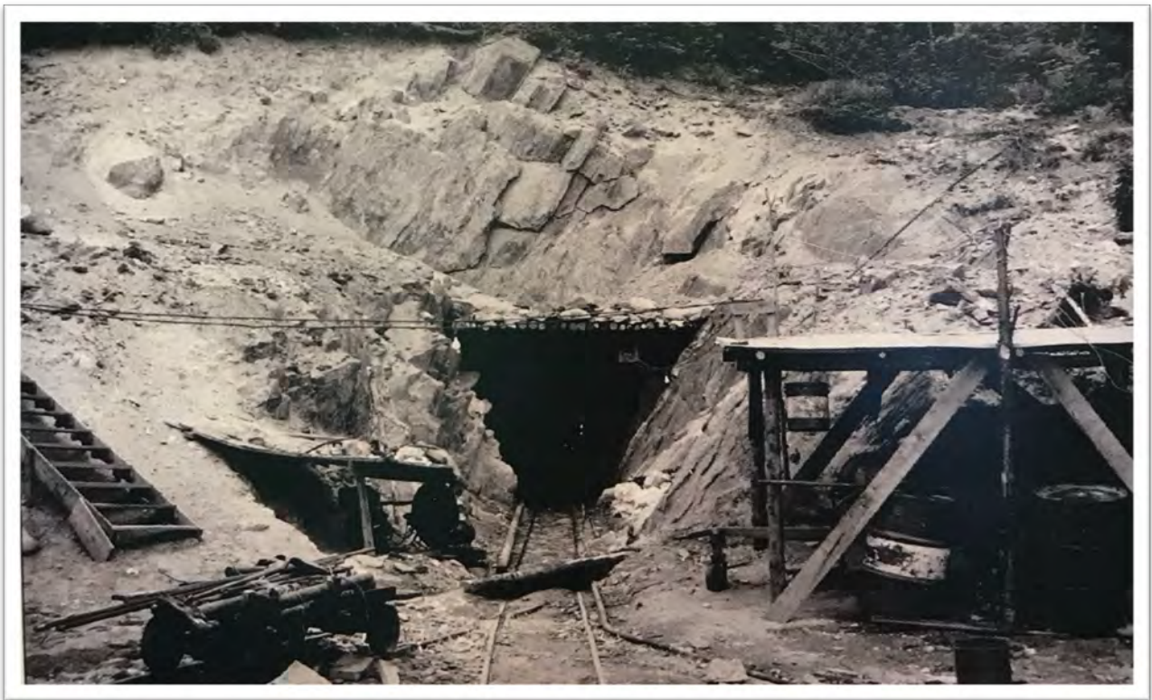
Switchback 4 mine in 1952
