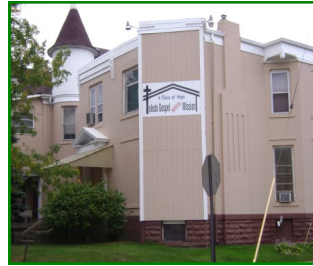
Men's Shelter 1917 Jefferson Ave.
