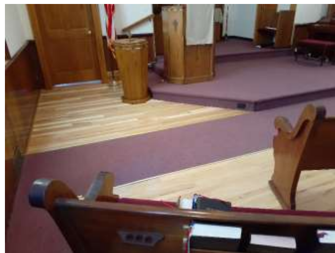
New flooring completed in the sanctuary provides greater accessibility.
