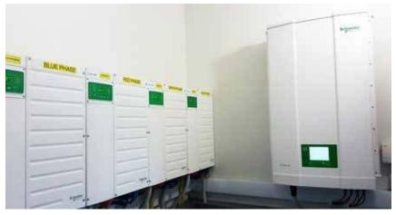
The multi-cluster is made up of 9 x 8.5 kW Conext XW+ inverters, which are all connected to a 5600Ah battery bank. In the battery room, a 20 kW Conext TL grid-tied inverter also manages the harvesting of additional solar energy
