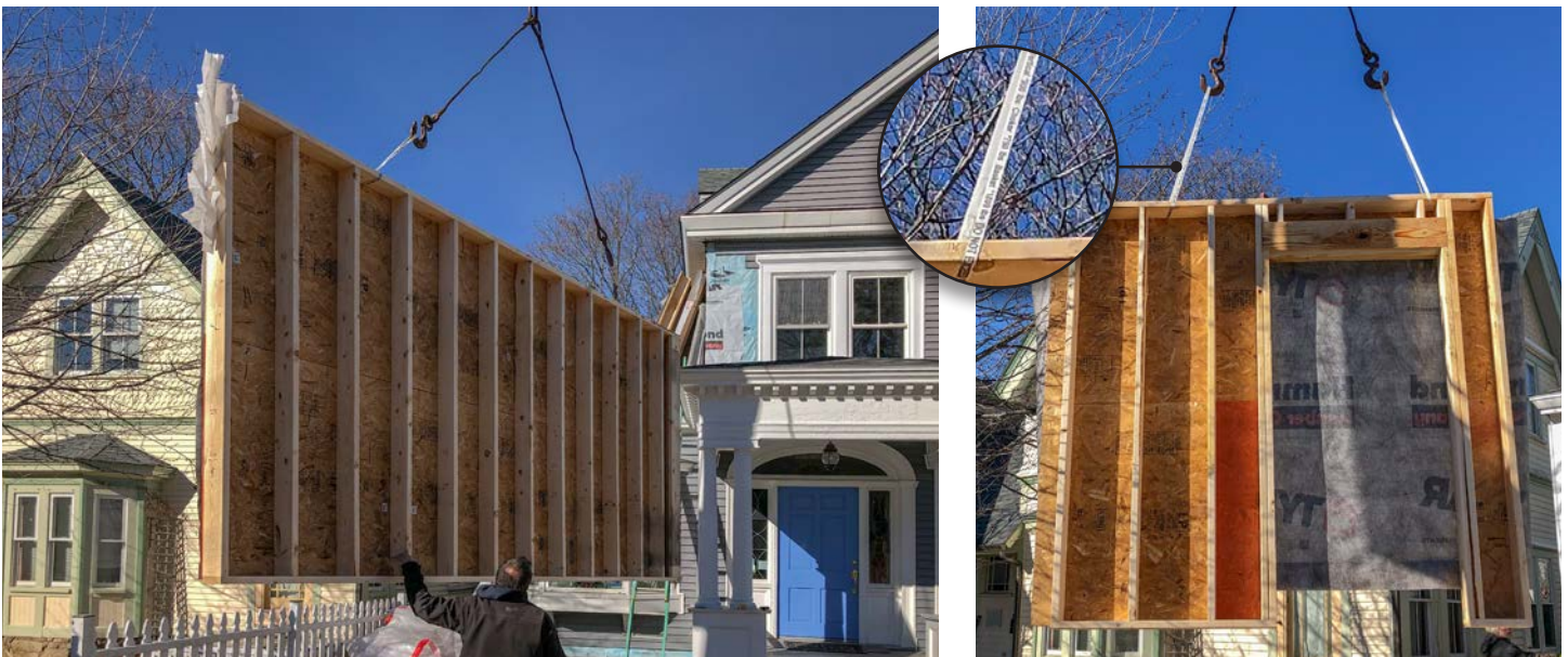
WALL PANEL LIFTING LOOP *Working Load Limit Vertical *900 lbs Choker *750 lbs Basket *1800 lbs DO NOT EXCEED WORKING
