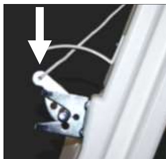
Step 4: Make sure gate latch catch is in down / locked position over striker bar. Extend string upwards to outside face of upper handrail & fold end approx. 1.5 - 2 inches. Mark handrail at fold in string for location of eye screw (see also Step 5 below)
