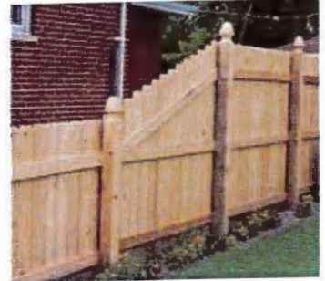
example of acceptable transition from 4' to 6'
