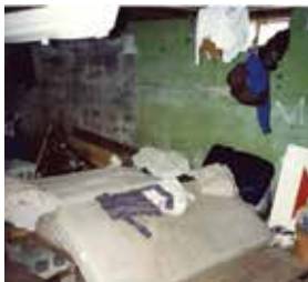
Inadequate Sleeping Area
