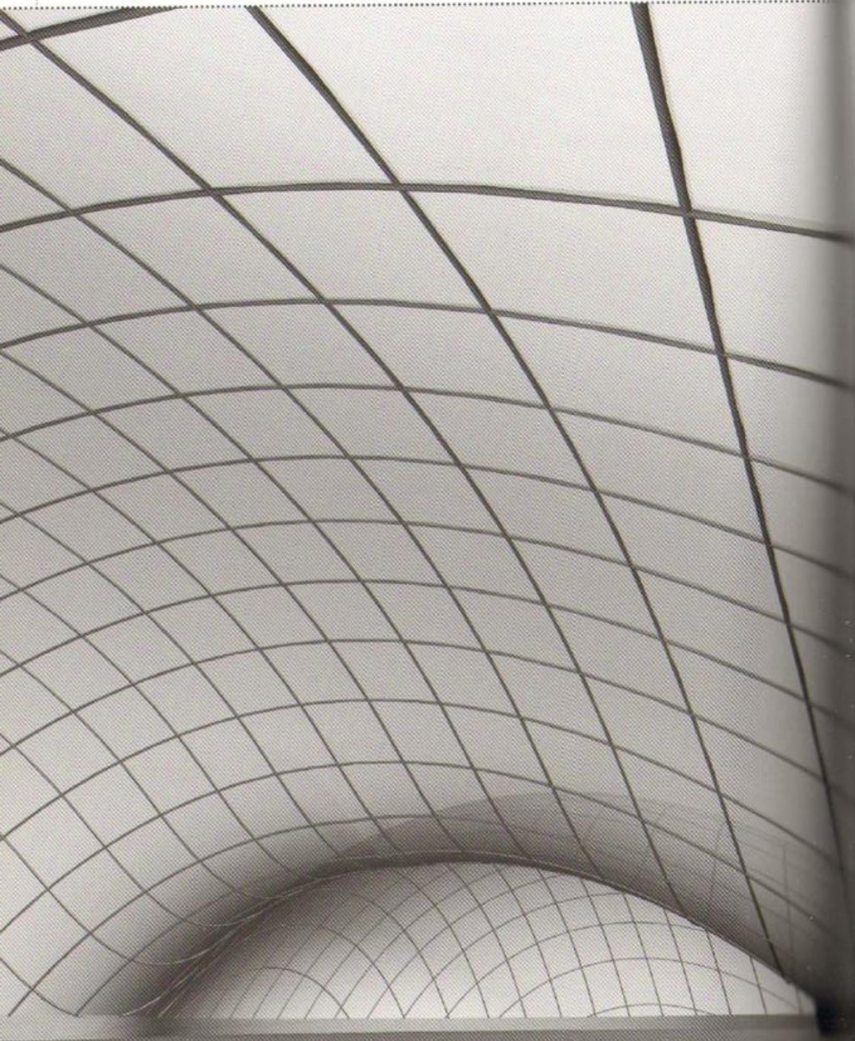
This curved form is produced by an air supported pneumatic membrane and a regular network of cables that consists of a regular grid spanning the perimeter and determining the scale of subdivision of the membrane as well as the curvature of the structure. This form transmits an optical affect of arching, quilting, amorphousness, rotundity and lightness, and an acoustical affect of focusing.
