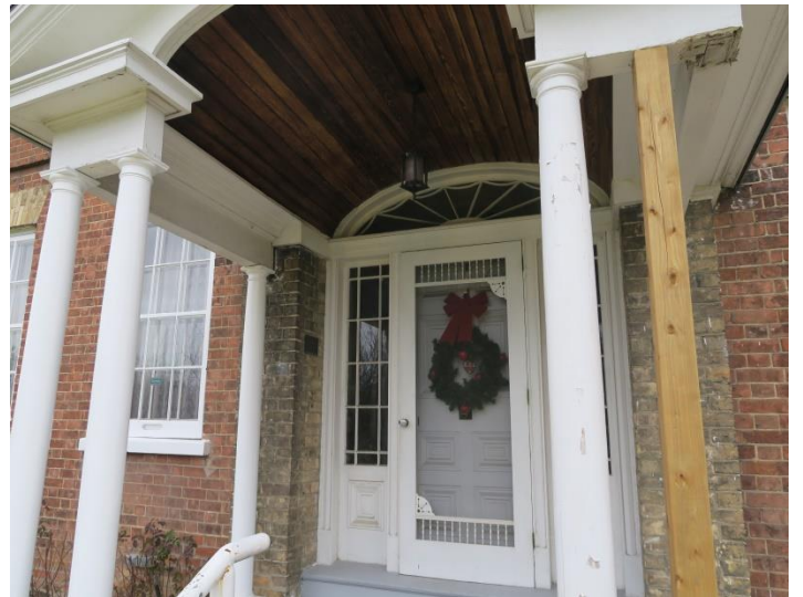
Deteriorated storms and delaminated pillars receive attention while COVID puts other Applewood summer events on hold. One-by-one, the front posts were removed, repaired, and repainted by Terry so that they could resume holding up the front porch for another hundred years!
