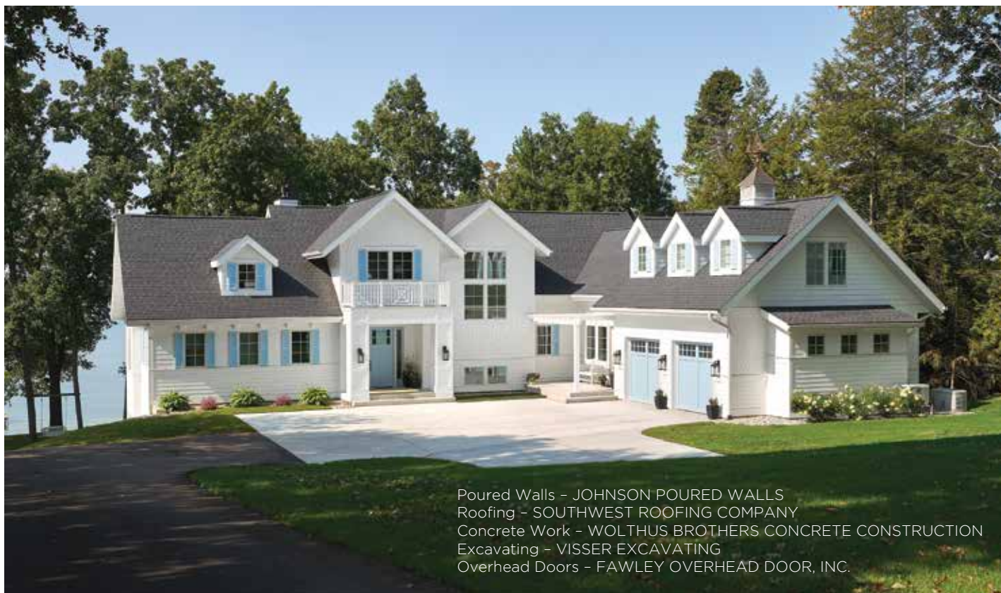
Siding - HVE INC. Steel Beams - OIK INDUSTRIES
