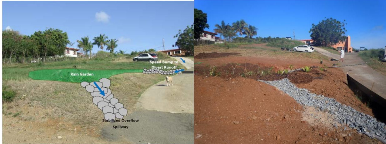
Figure 40. Initial rain garden concept (left) and finished rain garden (right), constructed as a part of a volunteer work day in October 2012.
