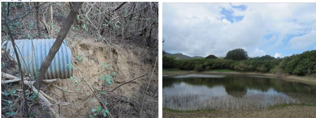
Figure 4. Large scour hole in the main gut, downstream of the 30-inch culvert under Pony Club Trail at entrance of Hope and Carton Hill (left). Further downstream, a large pond provides storage and habitat in the gut (right).
