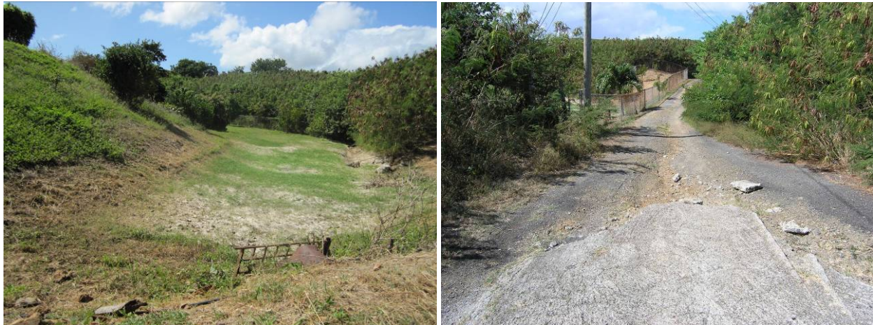
Figure 43. Gut downstream from large pond with two damaged/clogged culverts (left); the deteriorating road at the gut crossing (right).
