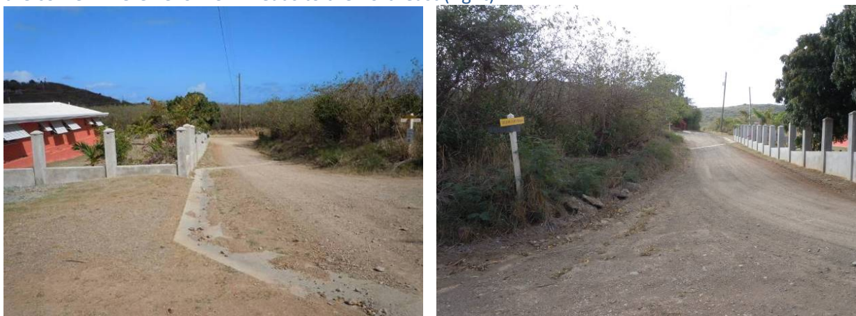
Figure 21. Shallow, paved swales at intersection with Hibiscus Circle (left), and the eroded ditch along the corner where Yellow Cliff heads to the northeast (right).
