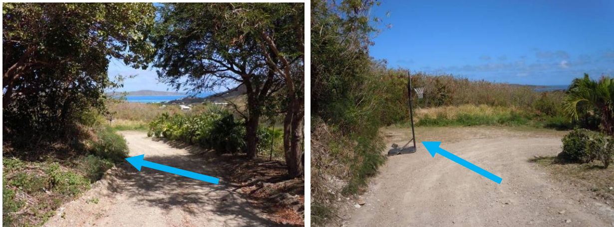
Figure 24. Runoff from the last portion of Ginger Thomas Trail flows to the western side of the road (left), towards the flat turnaround area where there were some signs of ponding (right).
