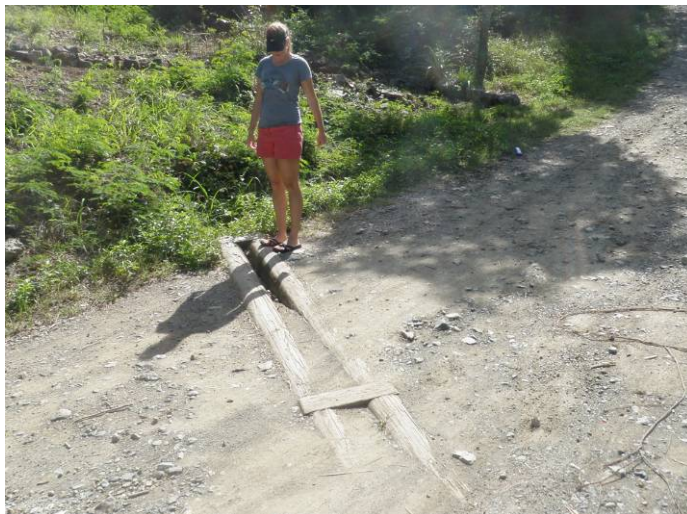
Figure 33. Open top-culverts have to be designed for maintenance access. The spacing should be wide enough to fit a narrow shovel. Top left and right photos here show clogged practices with reduced functionality. The grated cross-drain (bottom left) works on paved surfaces, and the grate can be lifted for easy cleaning. Be sure to provide outlet protection (bottom right) and remove deposited sediment on a regular basis.
