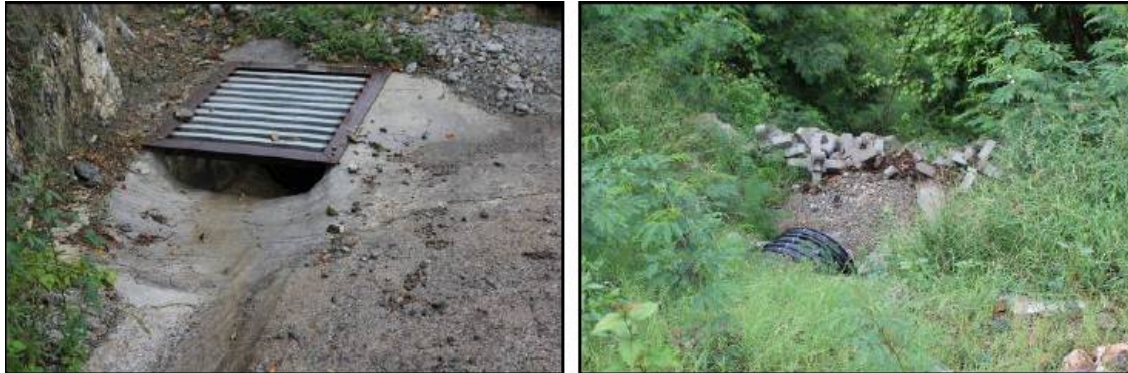
Figure 34. A drop inlet and culvert installed as a road improvement project in Coral Bay (Source CBCC).
