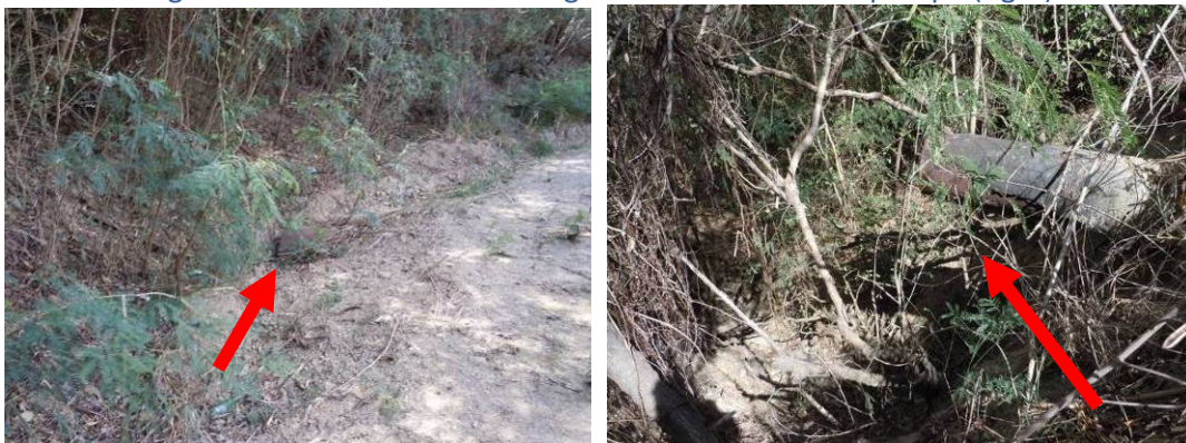
Figure 17. The upgradient end of the culvert is clogged with sediment, severely reducing its capacity (left), and the downgradient end has created a large scour hole on a steep slope (right).
