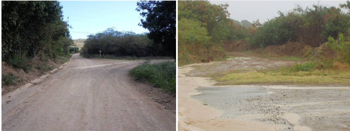
Figure 14. Shallow, paved swales at the downgradient end of Segment 4 (left), and a manmade drainage path created to help runoff reach the main gut – note piles of sediment exposed to runoff (right).
