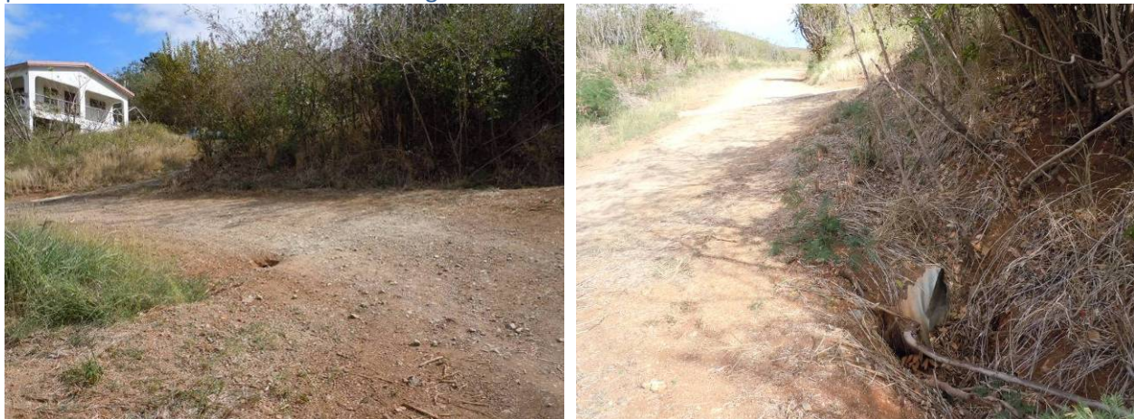
Figure 19. Clogged and damaged 24-inch corrugated metal culvert that carries runoff from the south portion of Hibiscus Circle across to the gut.
