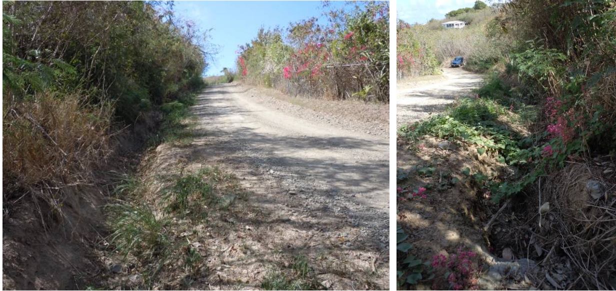
Figure 18. Looking uphill and downhill along the steep portion of this segment; the eroding ditch on the inslope is evident.
