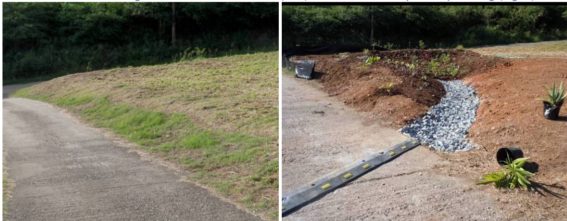
Figure 41. Before the rain garden was constructed (left) and immediately after planting (right).
