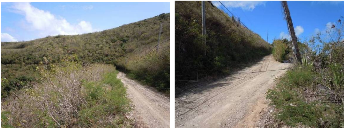
Figure 16. Yellow Cliff Trail is steep with an eroding ditch on the inslope.
