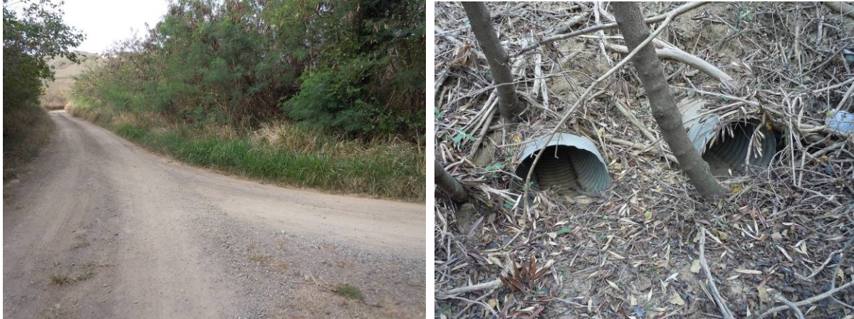
Figure 22. Portion of road that crosses the gut to the northeast (left), and the two 24-inch corrugated metal culverts at the gut crossing (right).
