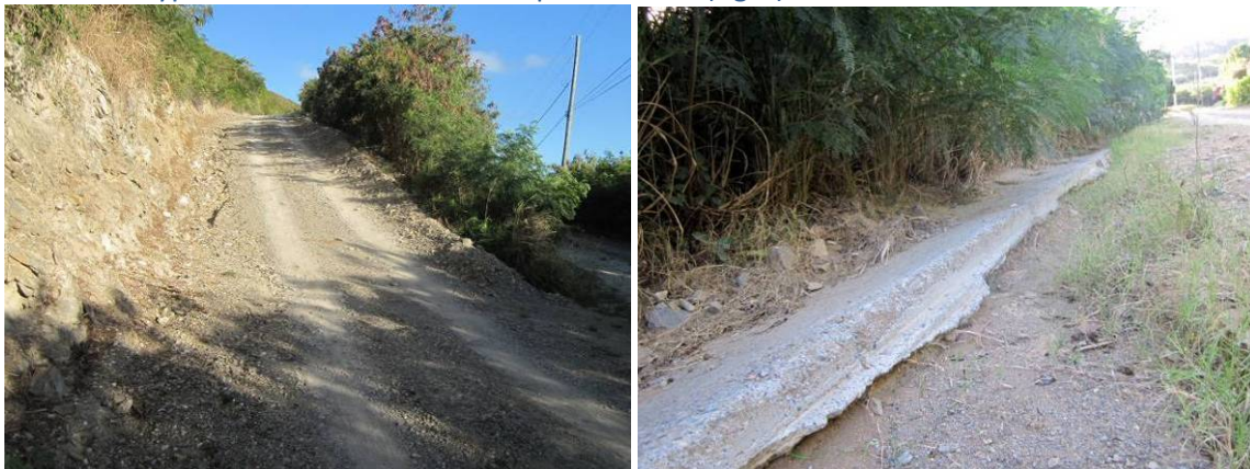
Figure 7. Roads in the Hope and Carton Hill Neighborhood are unpaved and very steep (left). Runoff from this road bypasses and undermines the paved swale (right).
