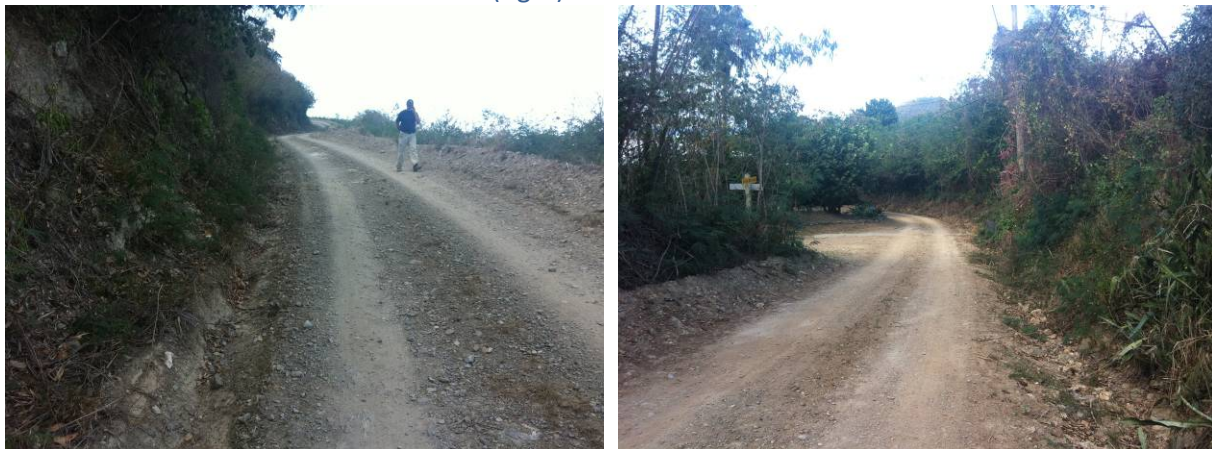
Figure 12. In some areas, the road has been graded down to the bedrock (left) with an eroding ditch on one side and earthen berm on the other (right).
