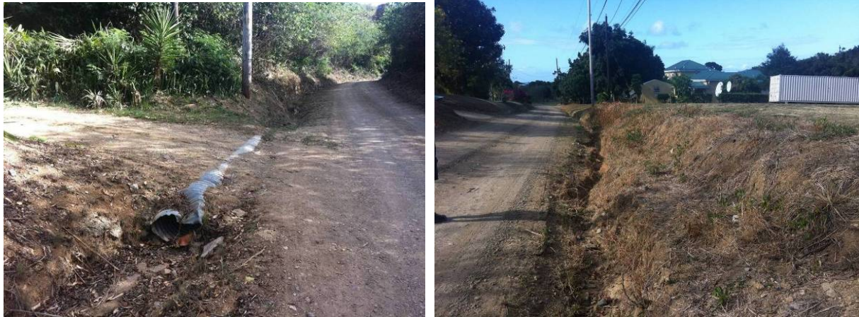
Figure 13. Damaged driveway culvert (left) and the eroding ditch serving as the gut (right).
