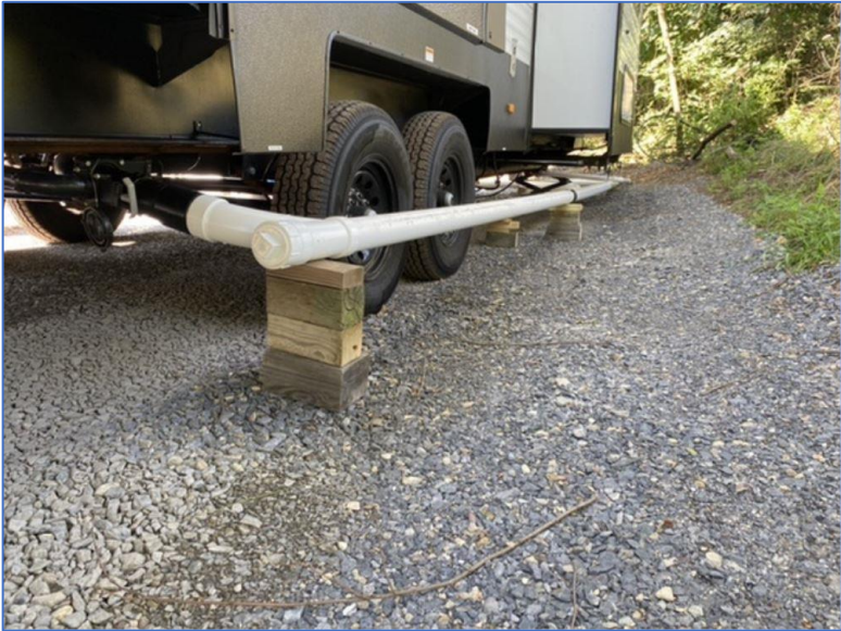
Sewer Waste Line Extension
