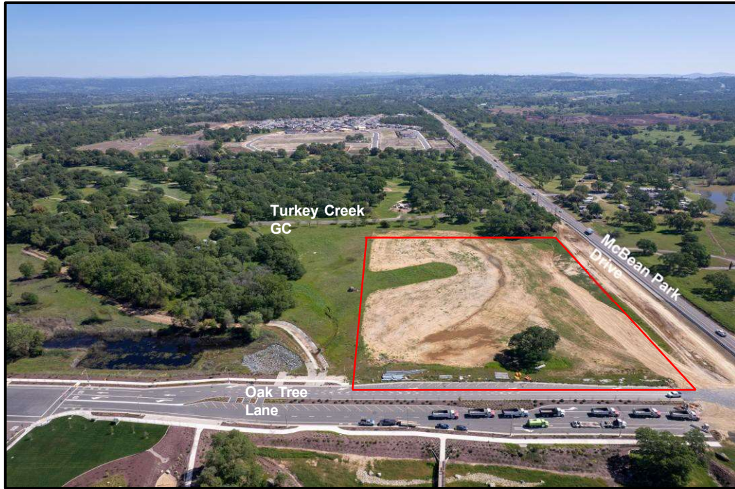
VIEW TO EAST
