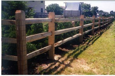
3-Rail Split Rail with green welded wire, locust post & hemlock rail
