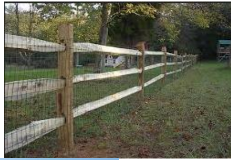
3-Rail Split Rail with green welded wire, locust post & hemlock rail
