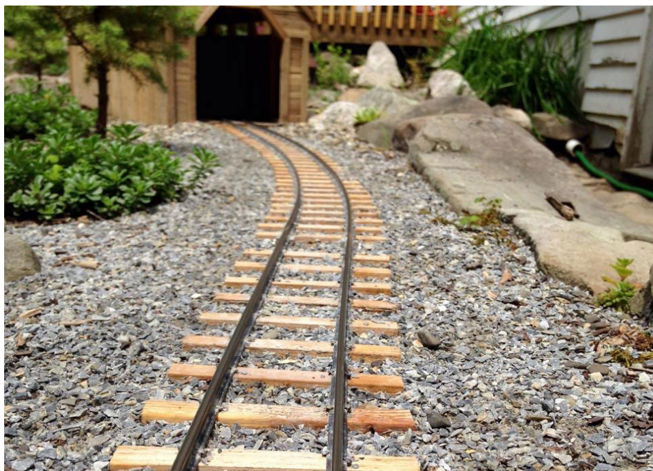
Hand laid track with cedar ties, newly laid above, is weathering well over the years.
